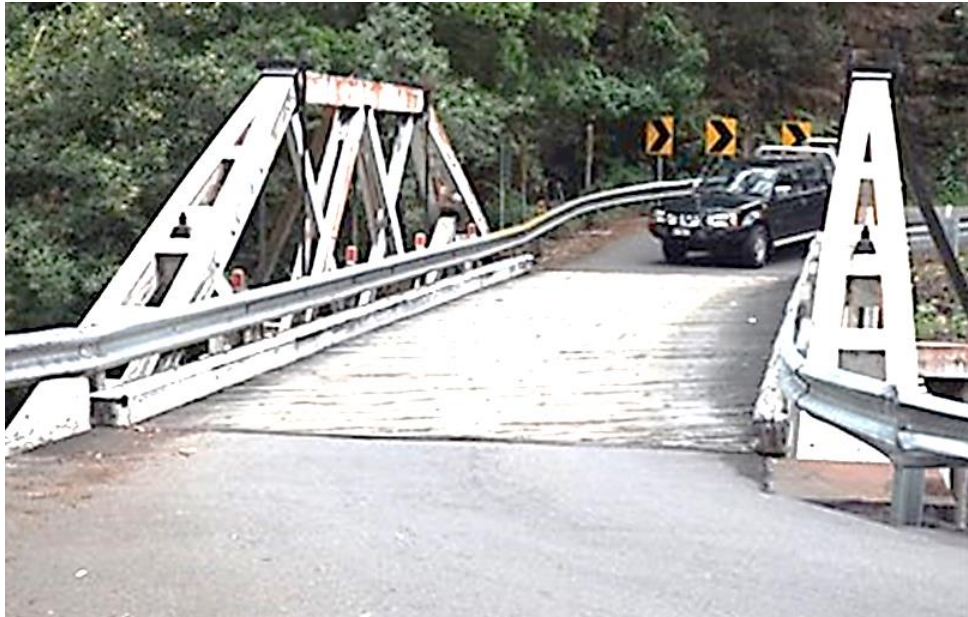
Image 46 (downloaded) - Here approaching traffic must wait for cars already on the bridge to pass before crossing. It's not wide enough for 2-way traffic.
